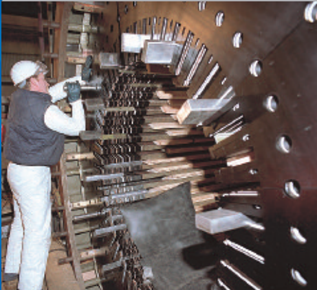
500 MW stator Core restacking
