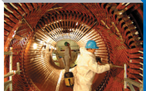
Replacement of stator coils on 1300 MW generator
