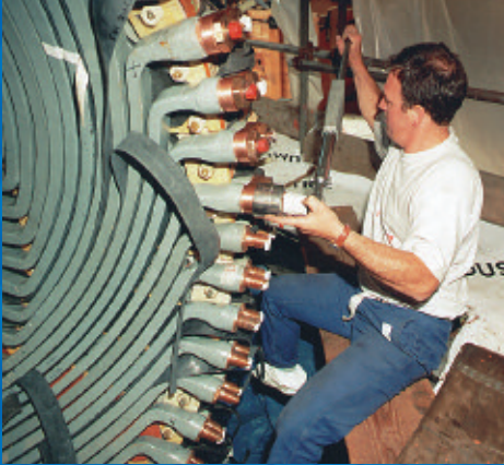
500 MW stator Core restacking
