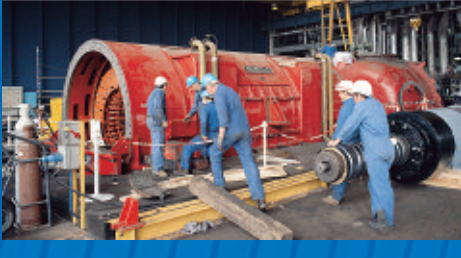
Removal of Jeumont 250 MW rotor end bells
