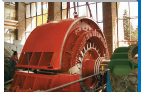
Replacement of stator coils on 1300 MW generator
