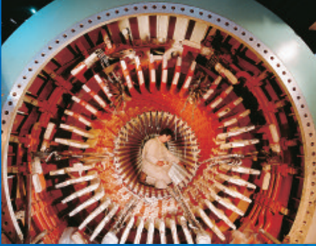
180 MVA generator overhaul
