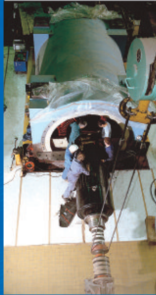
Reassembly of end bell on 80 MW rotor
