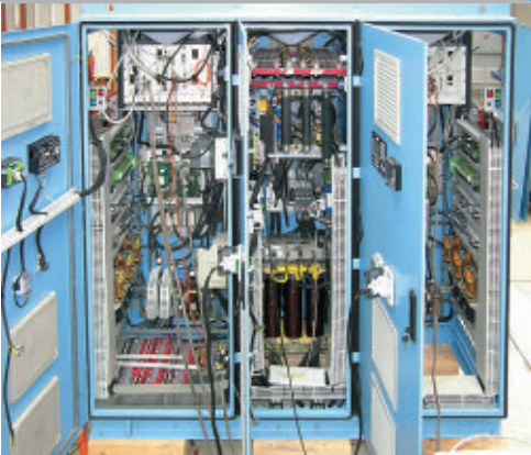
Test of AVR refurbished cubicle 900 MW nuclear plant
