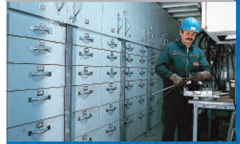
Overhaul area setup 900 MW generator
